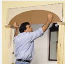
4. Slip columns on wall; rest template on top; draw arch shape.
