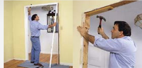
1. Remove existing casing in opening.
