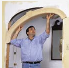
7. Slip arch header onto wall.
