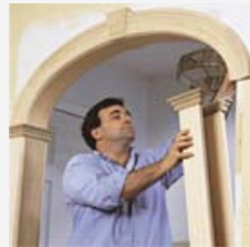
8. Slip arch columns under header.
