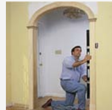
9. Level horizontally; nail all parts into place.
