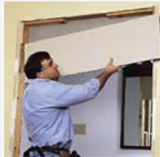
3. Cut a piece of sheetrock to fit top of opening and install.
