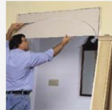
5. Remove existing sheetrock; patch.
