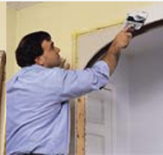
6. Apply sheetrock mud to seams and sand smooth.
